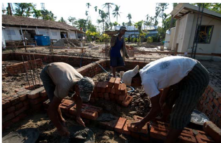
Constructing a health center, Kyae Chan Chaung Pyar village, ©IOM/Piers Benatar
